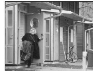
Figure 4 — The municipal housing authority in Lindås, Sweden, recently built 20 housing units that are so well insulated that heat from the residents, lighting, and appliances provides all of the space heating requirements.
